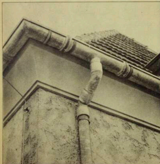
Rain Pipes and guttering are made of "Elernit," a substitute which saves metal . . . Iron railings are being removed from parks to assist rearmament.
