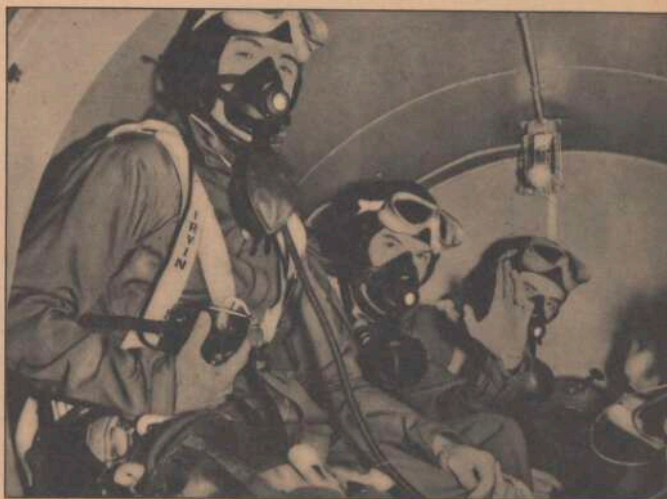
"Flight" These Denitrogenised Trainees enter strato-chamber for a 35,000ft. "flight." Even at sea level atmosphere, they must wear oxygen masks to avoid breathing more nitrogen. Each man wears complete stratosphere equipment, including emergency bail-out mask. This is attached to a small bottle of oxygen in a zipper pocket on his right leg. In stratosphere, necessary breathing pressure is automatically maintained by apparatus.
