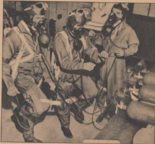
Oxygen Before Taking a stratosphere "flight" in Boeing strato-chamber, crews must exercise (above) for 30 minutes while breathing pure oxygen. This washes nitrogen—primary constituent of ordinary air—out of their blood. Bubbles of nitrogen in bloodstream at high altitudes causes aeroembolism—aerial equivalent of diver's "bends." This important problem involving lives of crews has now been solved.
