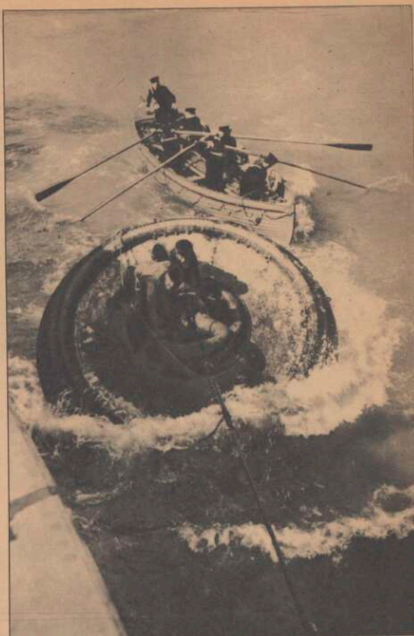
MOORING In Outer Reaches of many harbors, destroyers must be moored to huge buoys at end of convoy voyage. To make them fast safely, boat is lowered, two men climb on to buoy to fix hawsers firmly. In heavy seas, this is difficult job. Many new sailors have had unwanted swim at first attempt.
